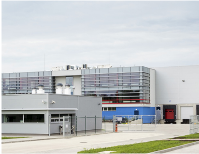
INDUSTRIAL AND MANUFACTURING
